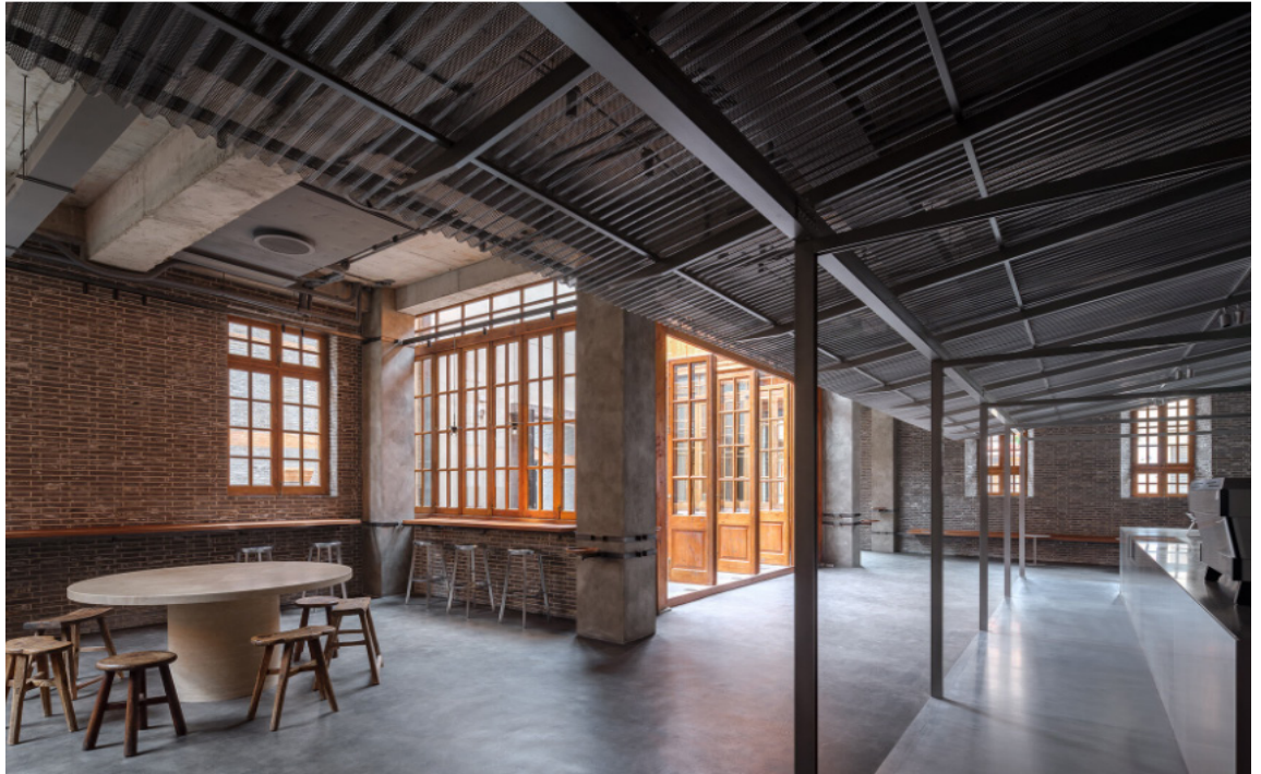
the original brick walls and timber framing are preserved
