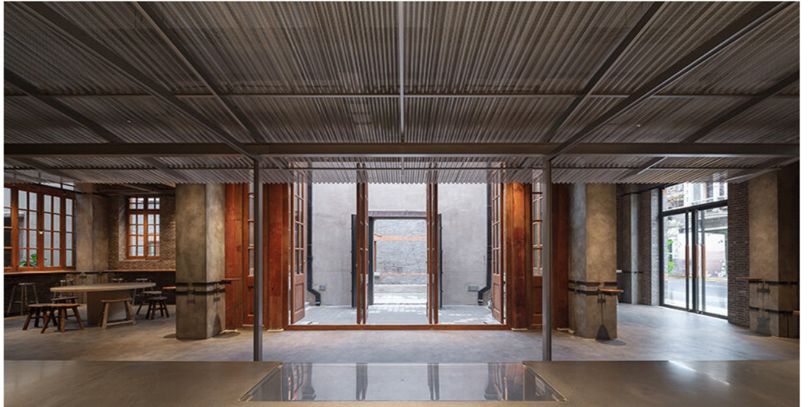
the roof of the shed is built of perforated, corrugated steel sheeting
